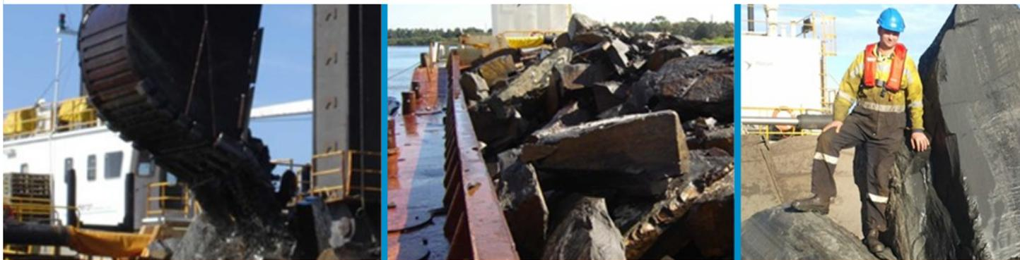
The backhoe dredge Machiavelli, along with 2 x 750m<sup>3</sup> and 2 x 500m<sup>3</sup> hopper barges and tugs Kurutai, Kotor and Nautilus were contracted to dredge 570,000m<sup>3</sup> of marine sediments, stiff clays and rock from the Hunter River for the new Kooragang Berth K10 for Newcastle Coal Infrastructure Group.
