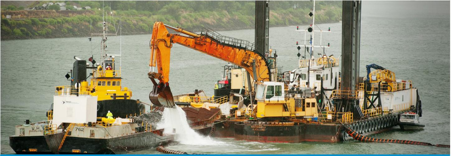
The backhoe dredge Machiavelli was used to dredge a combination of rock, stiff clays and marine sediments from the Hunter River for departure channel for the newly completed Newcastle Coal Infrastructure Group's Kooragang Berth K8 and K9.
