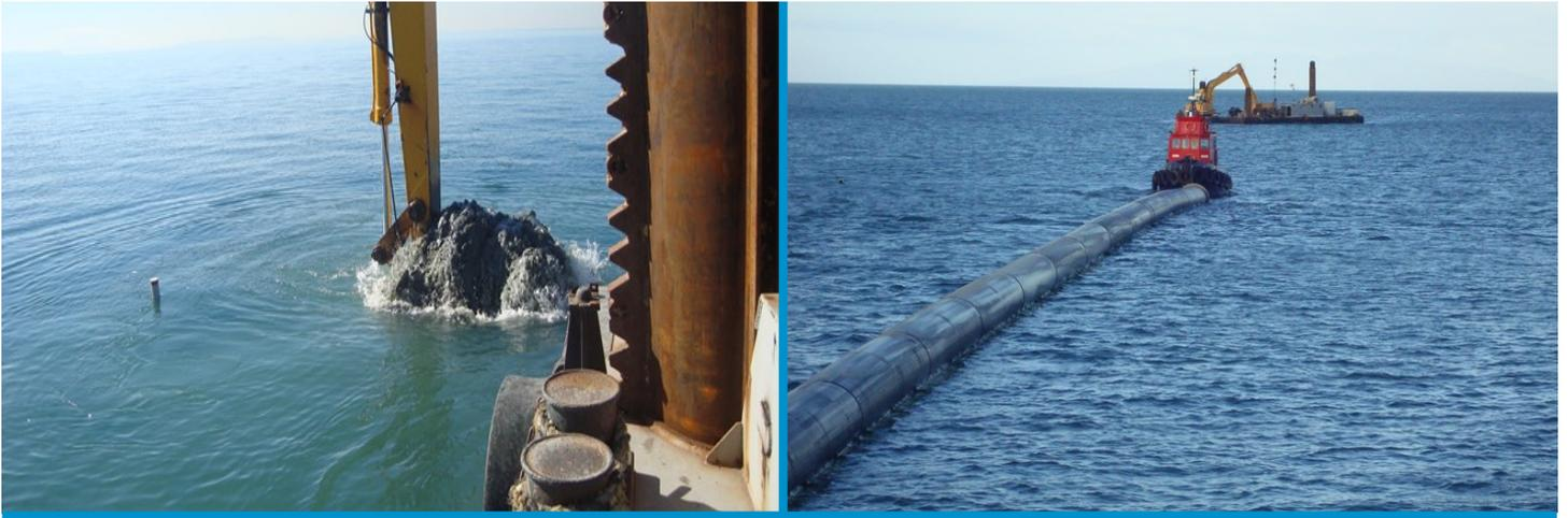
To protect and improve the quality of Auckland's beaches, a new tunnel and outfall was constructed allowing treated water from the Rosedale Wastewater Treatment Plant to be discharged 2.7 kilometres offshore into the Hauraki Gulf.
