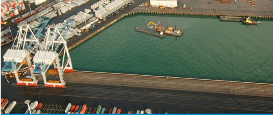
Heron Construction completed the dredging of 750,000m<sup>3</sup> of marine sediment, clays and sandstones from the Rangitoto Channel and the Fergusson Approaches and turning basin using the backhoe dredge Kimahia.
